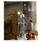
Chainfalls or other control means (e.g., procedures, micro-drives, load position/buffer) shall be used to avoid sudden overload of the crane or rigging gear. These lifts shall be treated as complex lifts.
